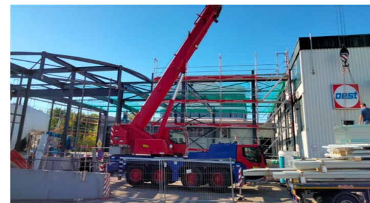
New building for empty containers at Georg Oest Mineralölwerk.
