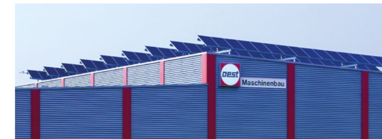
A powerful photovoltaic system is also part of the energy concept.
