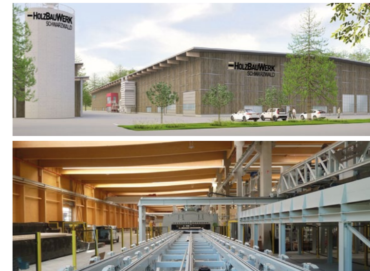
The new CLT factory in Seewald-Besenfeld, made of timber – naturally.
